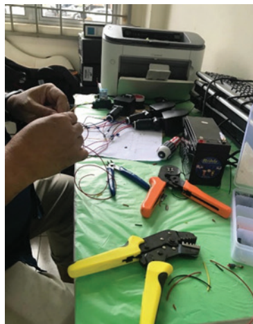
Figure 4: Wiring Installation Process
