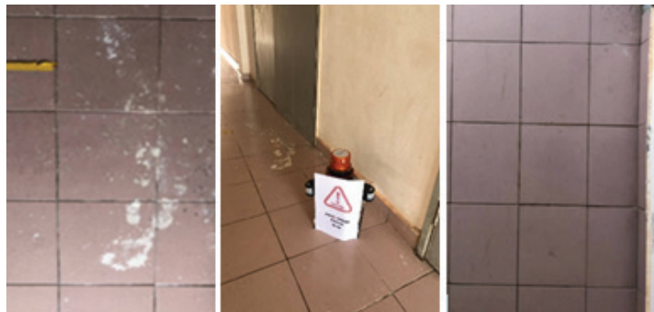
Figure 7: Before and After Installing Infrared Bird Repellent Sensor on the Sidewalk A
