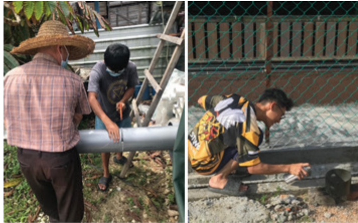
Figure 3: Cutting and Spraying PVC Pipe
